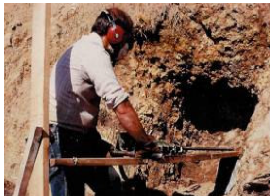
Figure 2. Drilling a Hole for Dynamiting
