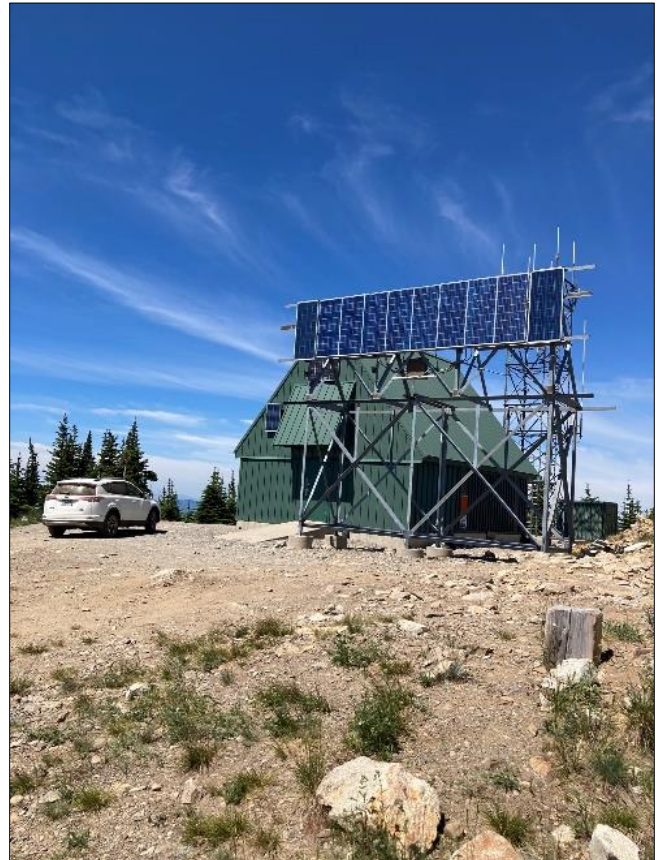
Figure 4. Buildings at Top of Peak
