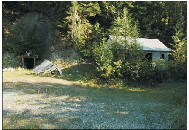
Figure 3. Mine office with main haulage adit to the left of center.
