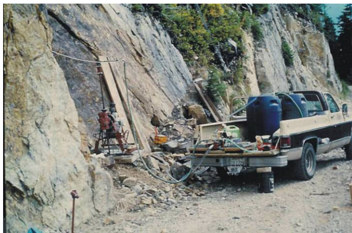
Figure 2. The Core Drill Setup
