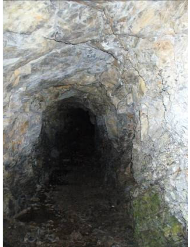
[The lower adit – either the Sunday or IOU mine.]
