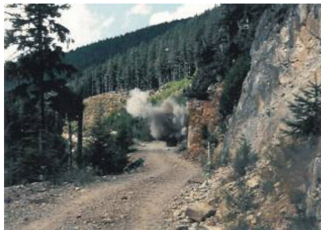
Figure 2. Blasting the Adit Entrance
