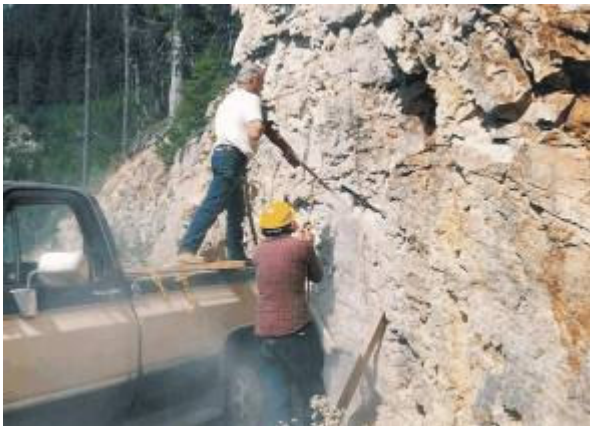
Figure 1. Drilling for the Adit Entrance
